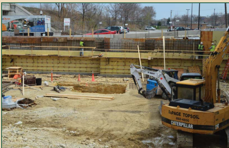
Forms are set for the front wall of the building. April 21, 2014.
