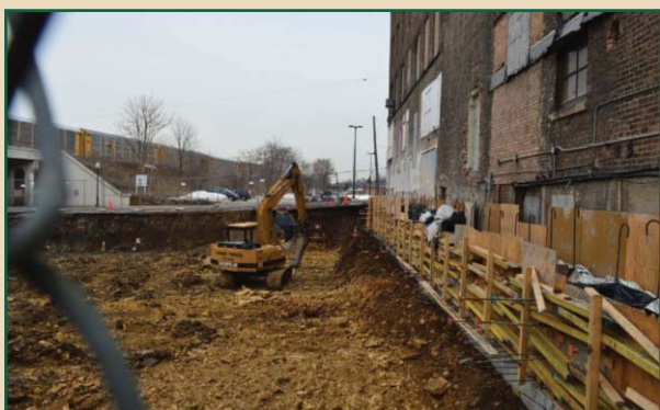
Digging out bedrock March 11, 2014.
