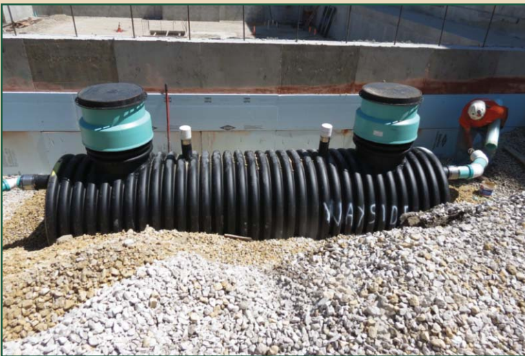
Grease Trap going in June 5, 2014.
