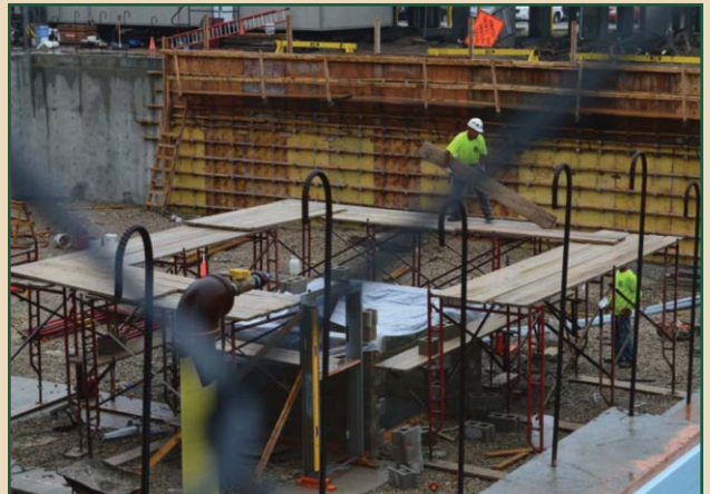
Front elevator shaft going up June 11, 2014.
