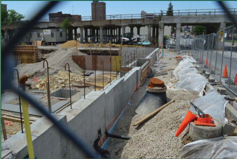
Back filling the front wall and under the side walk. May 28, 2014.
