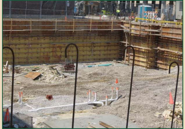
Plumbing is in, along with the stairway pad. June 2, 2014.
