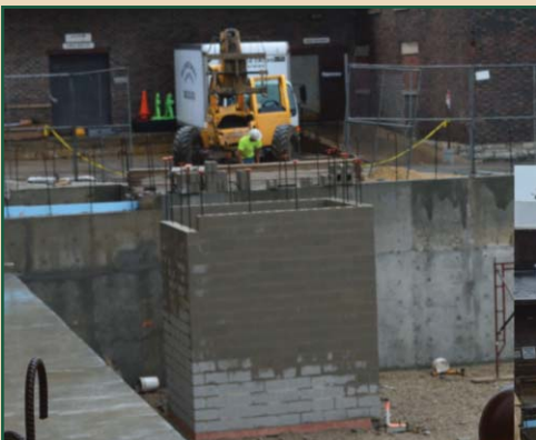
Back elevator shaft complete June 10th.
